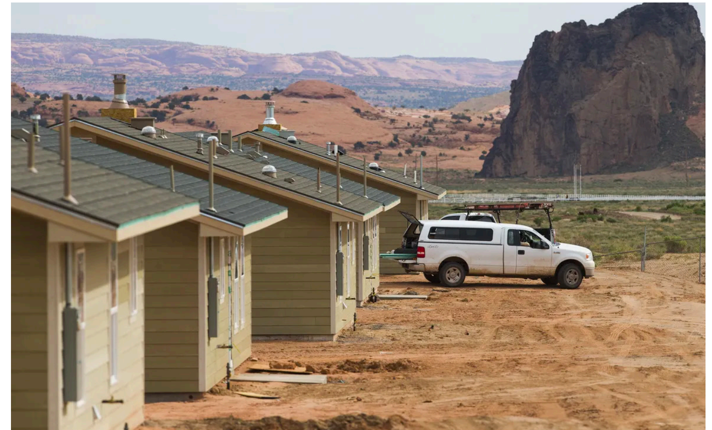
NHA Modular Housing Development in Kayenta, AR
